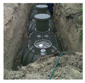
Devan septic tanks and underground vessels are made from an extremely robust grade of polyethylene specifically developed for use in underground products required to deal with the extraordinary forces of this type of installation.
