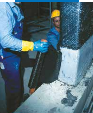
Application of MapeWrap onto the reinforced concrete element
