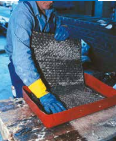
Manual impregnation of MapeWrap fabrics
