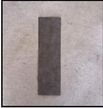
STEP 1: Cut a 200mm length of underlay at the same width as frames.
