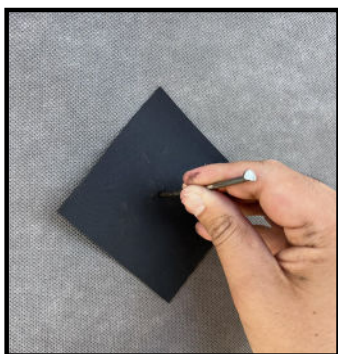
BLANK SEALS: Pierce blank FPS® Seal with a sharp point for each cable to pass through. Follow Step 2 & 3 above to ensure the seal is fitted correctly to the underlay.
