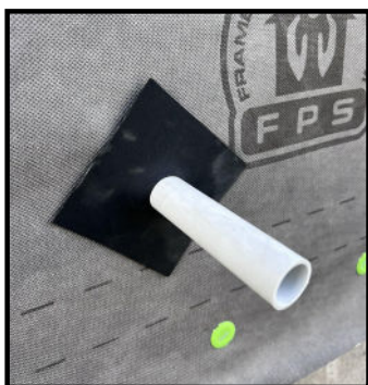
STEP 1: Install all FPS® Seals with a corner pointing up.
