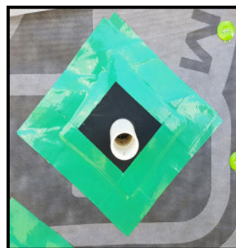
STEP 3: Remove the remaining section of backing paper and adhere to the FPS® underlay. Repeat for all other sides of the FPS® Seal, then firmly press tape with FPS® Spatula.
