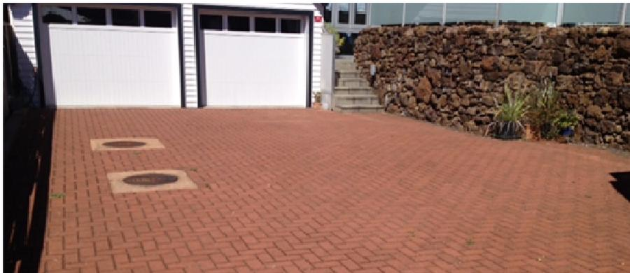
Figure 2-3 Typical Porous Paving used for residential application in Auckland (D&B Kettle Consulting Ltd 2013b)
