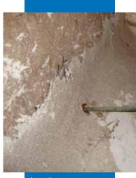
Inserting MapeWrap FIOCCO in the hole
