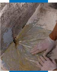
The splayed end of a piece of MapeWrap FIOCCO
