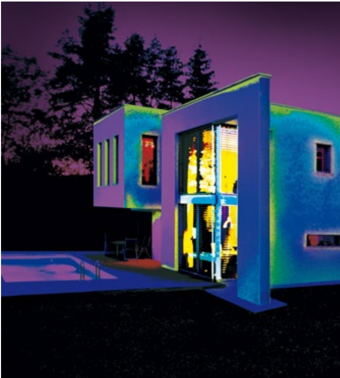
StoTherm insulation through thermography.
