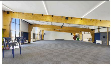
cut and fixed to the Glulam columns in our factory. A typical frame arriving on site consists of two Glulam columns with gussets attached and one continuous pitched rafter member. The rafter is able to extend beyond the columns thus providing an overhang. For large spans the rafter can be supplied in two sections with an apex gusset. All members are pre-finished in factory and require no further attention once erected in industrial buildings.
