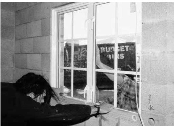
A: Once the window is fixed and square install backing rod and foam airseal to the interior of the joney.
