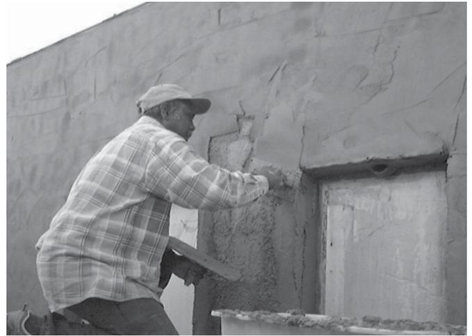
it makes a slight hollow sound. After this preparation coat, it is common for two or three coats of plaster to be trowelled on. It is even possible to spray the plaster on which speeds up the process. The top coat of the plaster can be coloured to match the paint just like an undercoat.
