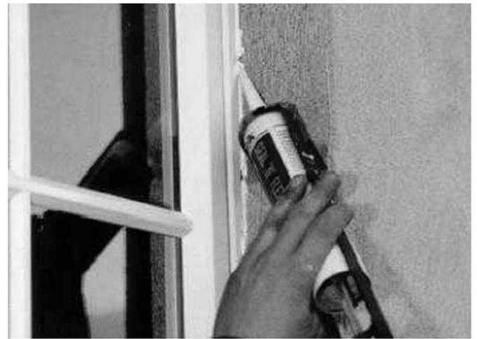
B: apply a flexible seal to the gap between the top and sides of window frame and masonry wall. Do not seal along the bottom of the window frame.
