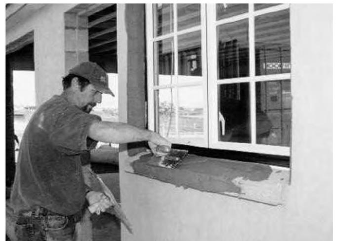
With the paint system, it is very important that the paint coat is applied over the flexible sealant up to the joinery. This provides one extra defence against moisture ingress. The Architect or Designer should fully detail the weatherproofing procedures for window openings.
