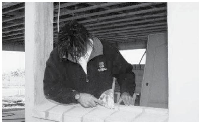
Apply a waterproofing membrane around head, jambs, and sill. This waterproofing membrane should cover the entire thickness of the wall and be extended a minimum of 50mm on the exterior face around the penetration.
