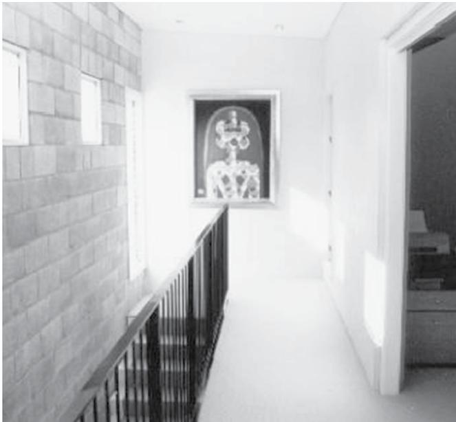
Paint over bare blockwork is a relatively low cost solution. This provides a uniform colour to the wall and still allows the mortar joints to be seen. It is important that the walls are as dry as possible before applying the paint. If any excess moisture is trapped, it is likely to bubble the paint over time. In order to hide the block lines, a high-build elastomeric coating with a levelling coat can be used.
