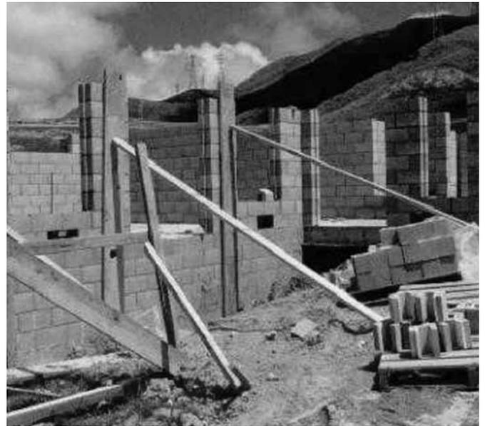
Typically bracing at 3m centres is recommended in line on both sides of the wall.
