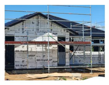
IBS RigidRAP®-XT should always be installed vertically with the arrows pointing upwards when installed as a bracing element.
