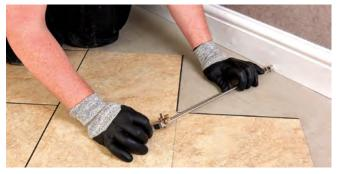
Figure 4.9 Cutting the tiles using a scriber (diagonal cut)
