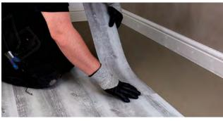
Figure 5.1 Setting planks out
