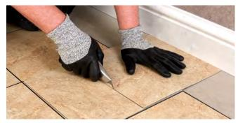
Place the tile to be cut exactly over the last tile laid, ensuring the colour is correct and the decoration runs the correct way.
