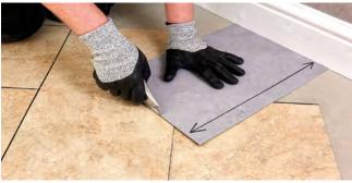
Figure 5.9 Cutting the perimeter tiles (diagonal cut)
