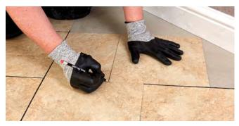
Figure 5.8 Marking using an overlapping template on diagonal laid tiles
