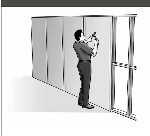
Figure 4: Fixing remaining sheets
