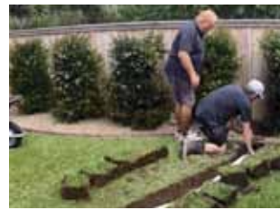
3. Lay QuickDrain
