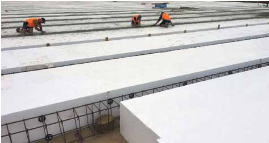
EXPOL GeoFoam as lightweight fill under a concrete floor
