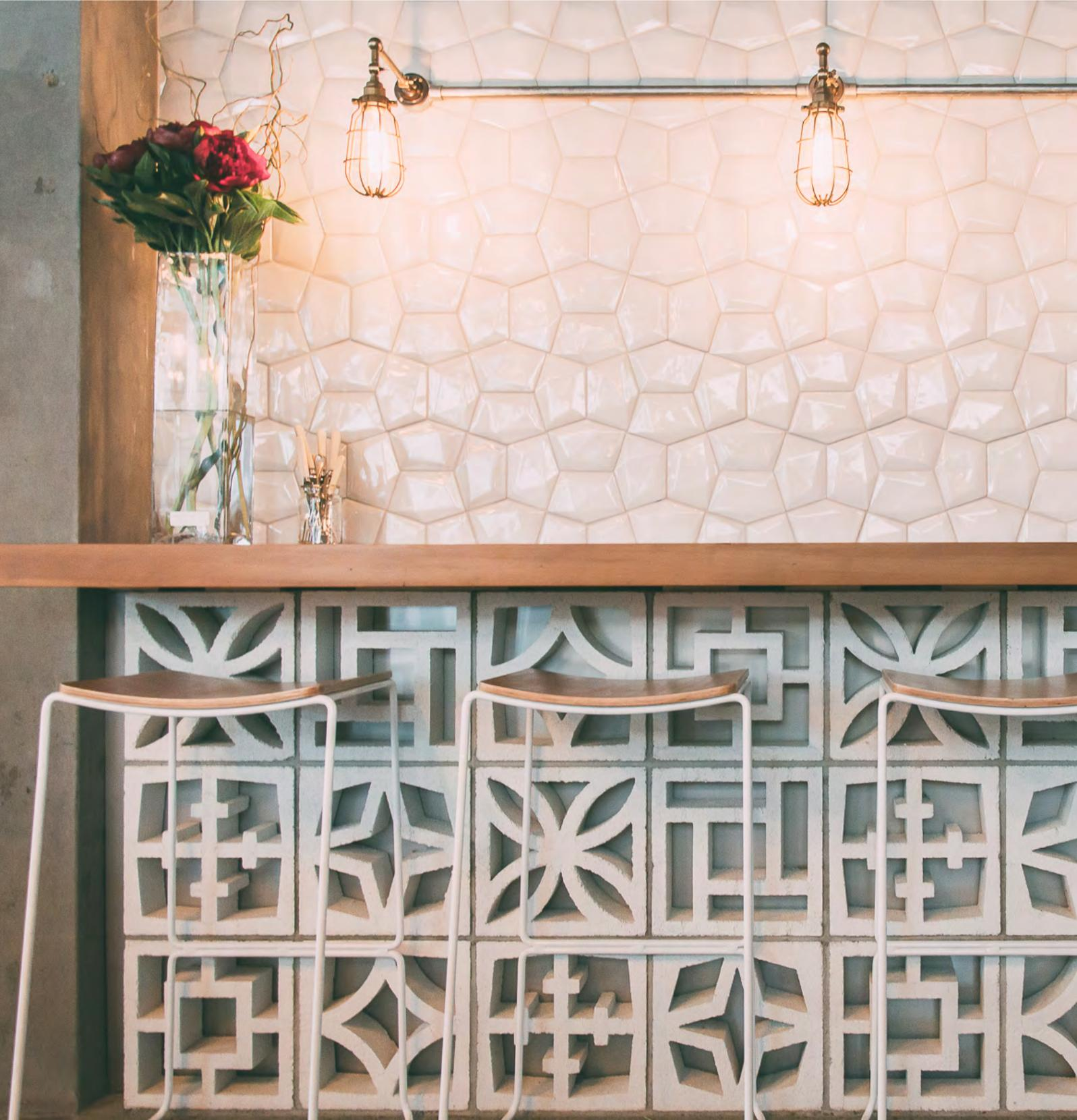
**Firth Solar Screen Blocks have a decorative open pattern through the face of the shell allowing the breeze to pass through and provide shade from the sun.**
