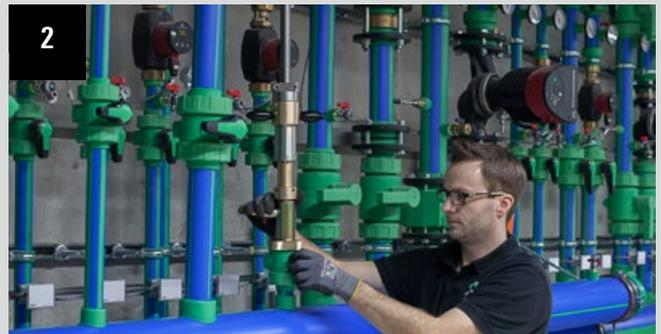
2. Assembly of the hot tapping tool onto the component
