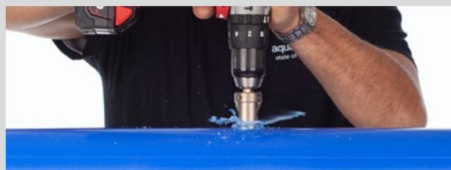
Drilling through the pipe wall
