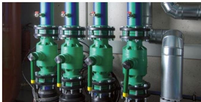
Risers and distribution piping for heating supply should be planned and installed with aquatherm blue pipe fibre composite pipes.
