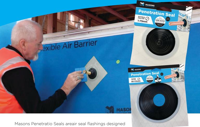
Masons Penetratio Seals areair seal flashings designed for cavity construction where pipes or wires penetrate building cladding and pass through the air seal membranes such as synthetic building wrap, or a flexible or rigid air barrier.
