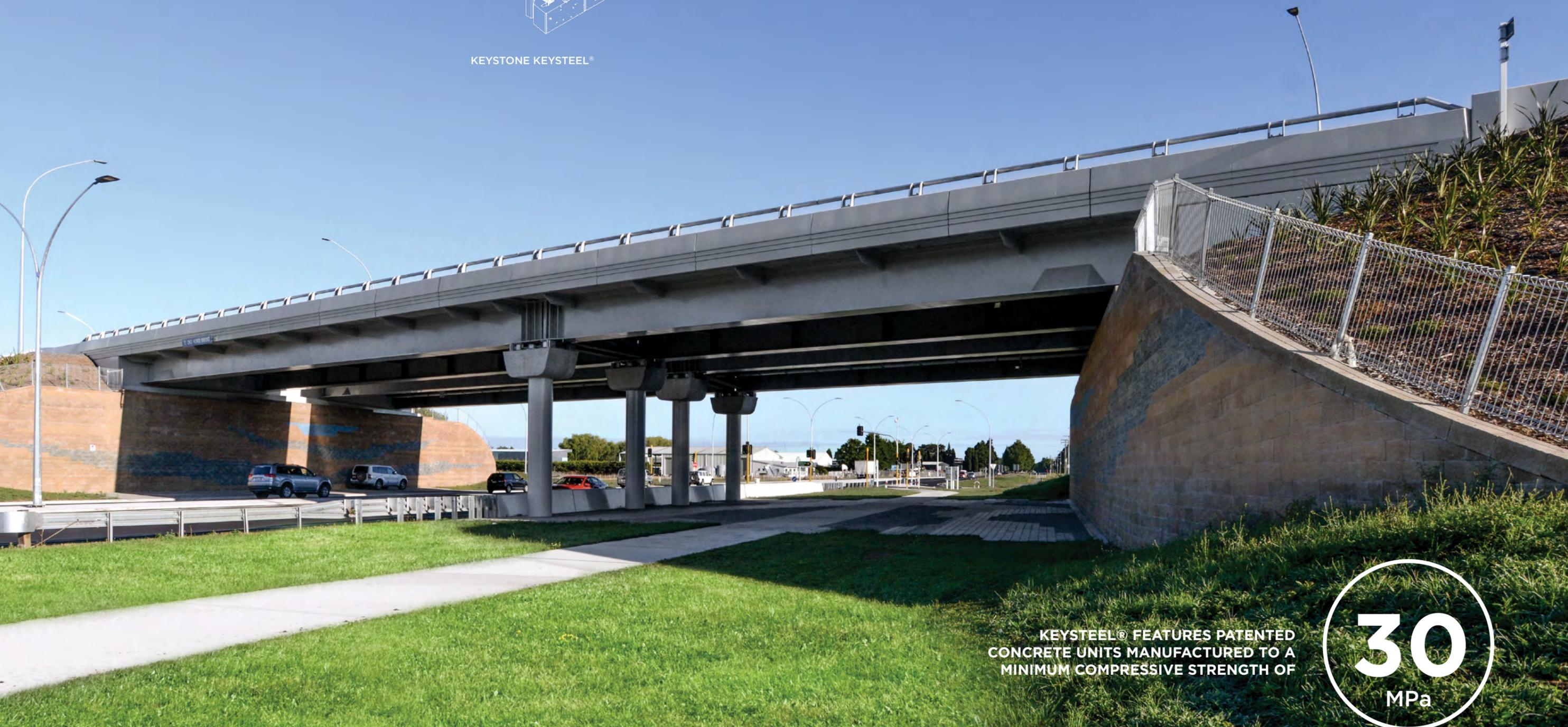
KEYSTEEL® FEATURES PATENTED CONCRETE UNITS MANUFACTURED TO A MINIMUM COMPRESSIVE STRENGTH OF
