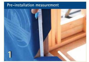
Measure vertically up the jamb from the internal corner of the sill. Minimum 100 mm allowing for 50 mm cover onto the wall underlay.
