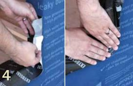
Remove second release foil to allow for application onto weathertightness layer.
