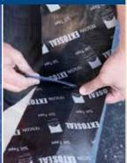
Remove first release foil to allow for application onto sill and jamb framing. Start installing the Sill Tape from the first preinstallation measurement of the first jamb.
