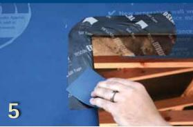
Measure vertically down the jamb and horizontally across the head trimmer from the internal corner. Minimum 100 mm allowing for 50 mm cover onto the weathertightness layer. Repeat installation to jamb and head trimmer as per steps 3 and 4.
