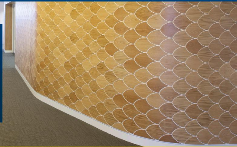
Gyprock Flexible is a 6.5mm plasterboard sheet with an enhanced gypsum core in a heavy duty liner paper that enables the board to bend to a small radius.
