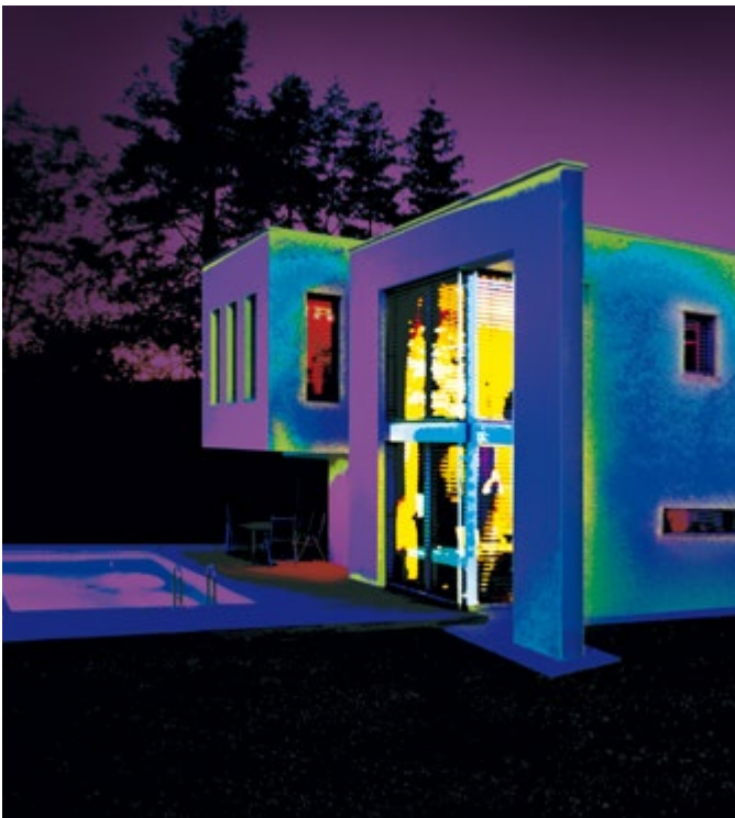
StoTherm insulation through thermography.
