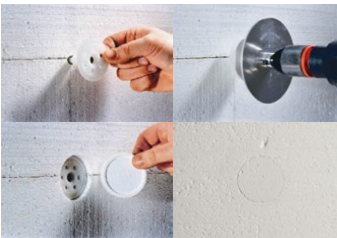
StoTherm Anchor installed on timber frame.
