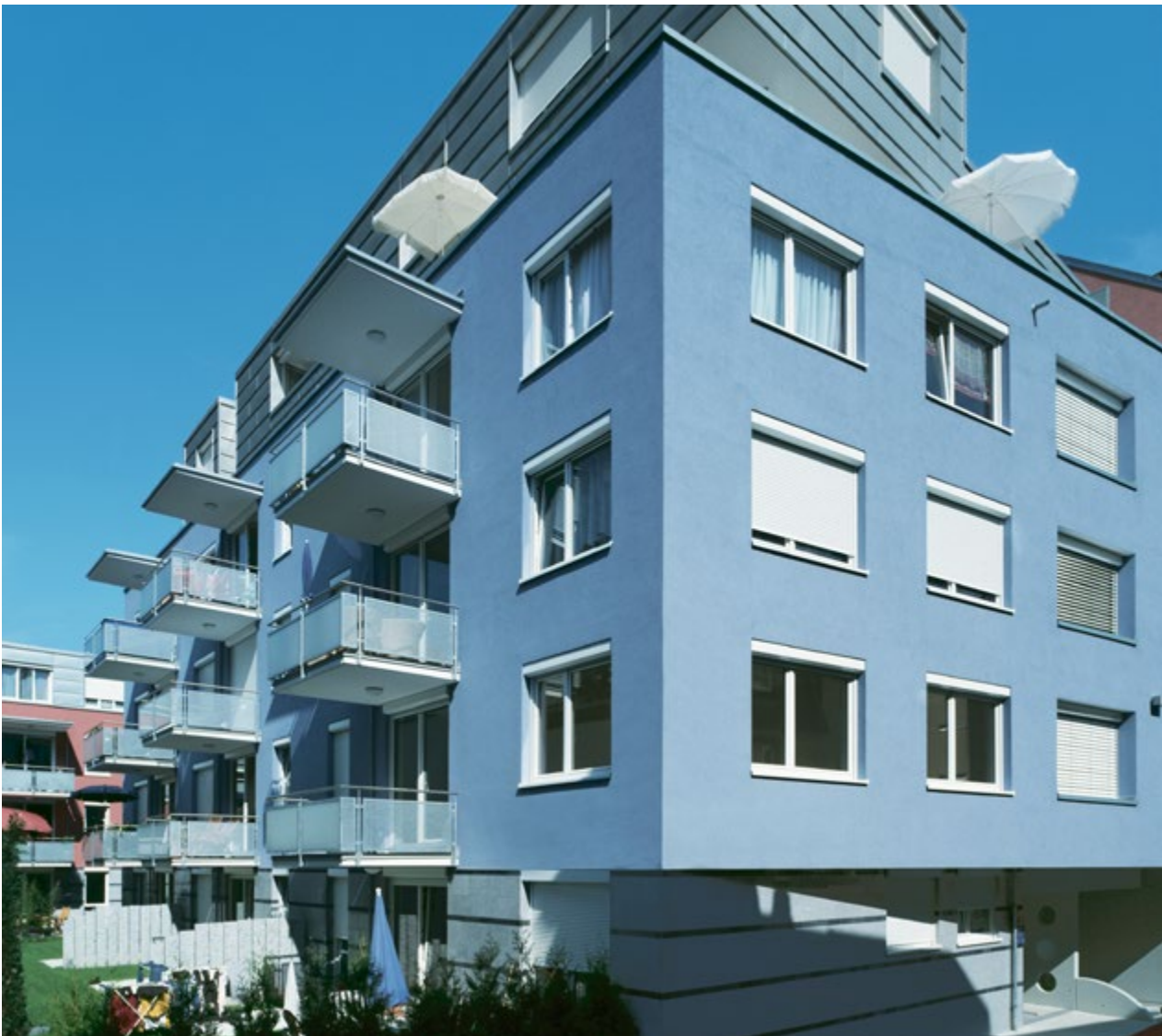
StoTherm: New build Residential, Offenburg Architect: Dipl.Ing. Koger, Krongutstr.
