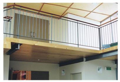
underside has "V" shaped edges and is filled and sanded to provide a complete ceiling system.
