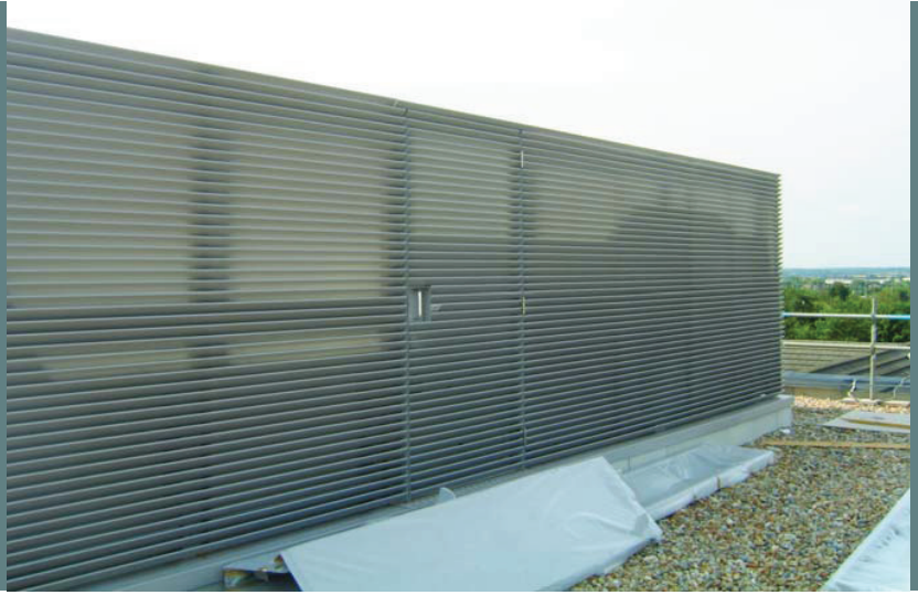
William Harvey Hospital, Ashford. 1UL/SH inverted louvre panels.
