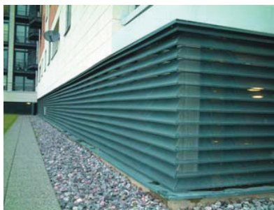
Perforated louvre allows additional daylight into this partially underground car park.
