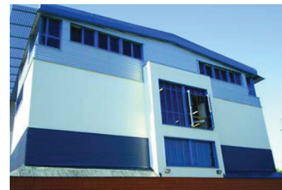
Crawley College, Crawley. ERD louvre panels on the plant room, and Solarfin solar shading panels.
