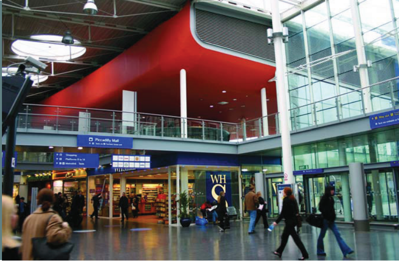
Piccadilly Station, Manchester. A combination of single and double bank louvres, depending on the specific airflow and rain defence requirements.
