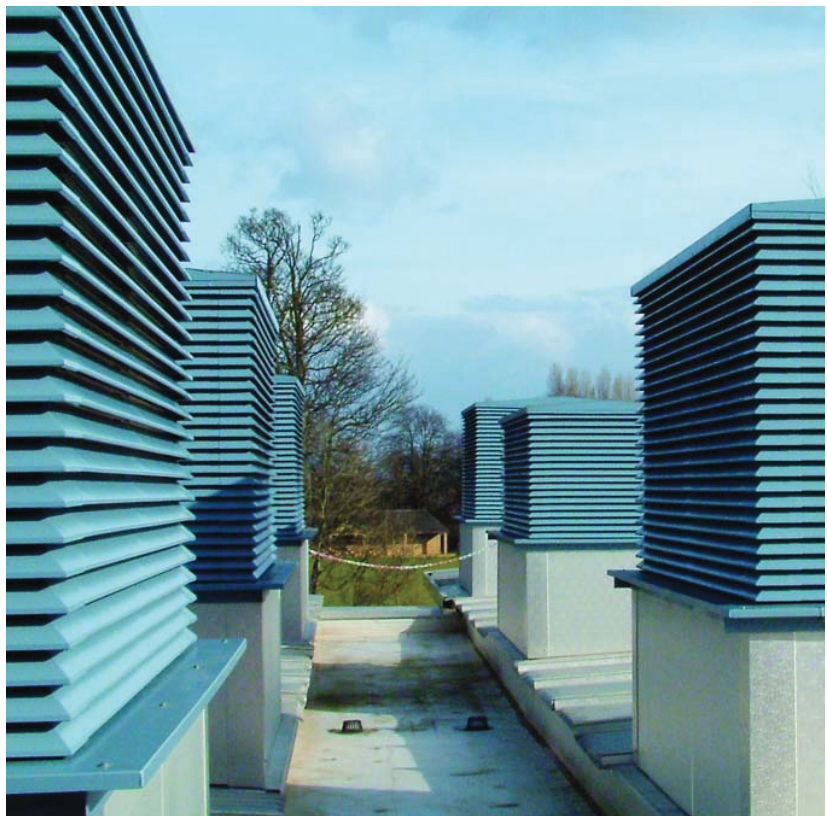
Portway School, Bristol Pre-assembled 3UL louvre turrets on top of natural vent shafts.
