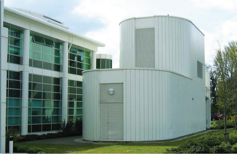
National Physical Laboratory, Teddington. 1UL/SH panels with upgradeable 2UL/SH panel sections.
