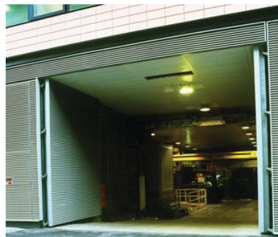
UCL, London. Louvre doors to loading bay.
