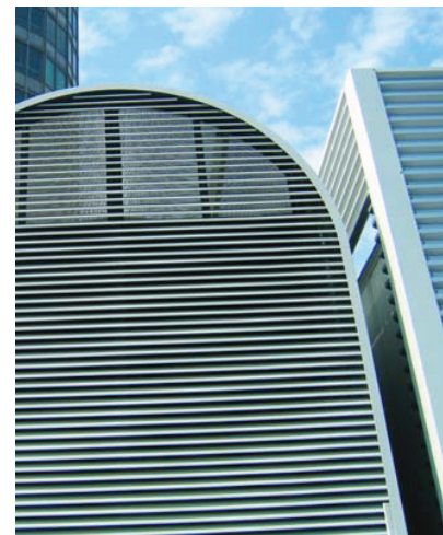
Arup Fitzrovia, London. 2UL rain defence screens for plant rooms.
