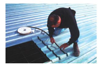
Furthermore, gaps in the pans of dissimilar materials can occur. The foam tapes fill up these spaces much more effectively than silicone. The end lap fixing methods are the same for metal onto fibreglass, fibreglass, or fibreglass onto metal.
