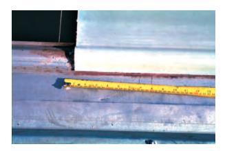
At all end laps two lines of compressive foam strip or of flexible sealant shall be placed across the full width of the lap approximately 150mm apart and with one line 25mm from the end of the Fibreglass sheeting. Ampelite recommends the use of foam tapes rather than silicone. Silicone sealants tend to bond the two end lapping sheets together preventing individual sheet movement.
