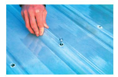
It is important not to over tighten the screw putting undue pressure on the fibreglass sheet. 32mm "Weatherlok" seals are large enough to cover the oversize hole and are sufficiently flexible to contour to any corrugation when medium pressure is applied. Medium pressure means that the "Weatherlok" seal is contoured to the shape of the rib but the rib must retain its shape without any sign of buckling. (Note the washer on the top is too tight, the washer on the bottom is OK.)
