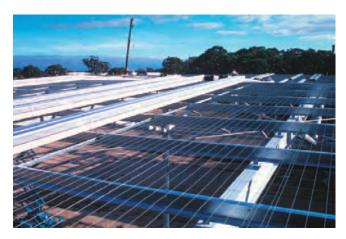
Protective Pulin Strips are available from Ampelite, in the following sizes, in packs of 10. The strips have double sided tape on one face to help hold them to the prulin until the fiberglass sheeting is installed.
