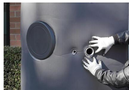
Ensure the drain is fitted or plugged. Ensure the tank is in position where it's going to be installed, as it can be difficult to move once the insulation is attached.
