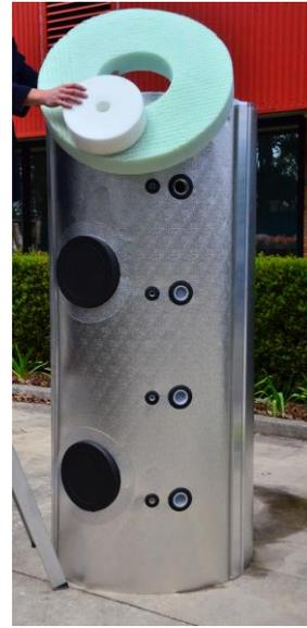
Continue using the same process to wrap each panel around the tank. Once all panels are joined each panel should be tightened into the last tooth if possible. Ensure the teeth are fully engaged along the entire length.
