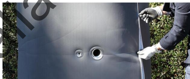
There are 14 plastic fitting surrounds, these vary in size and should fit tightly around the fitting. The fitting surrounds are placed on after the insulation and should sit flush with the front of the fitting. Attach the fitting surrounds as each section is put in place, this will help to hold the section in the correct position as each is added.
