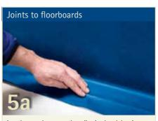
Lay the membrane on the adhesive bead, leaving an expansion joint and do not press the glue down completely to allow for differential movement at the joint.
