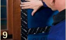
Seal the wall wrap to the joinery using the TESCON EXTORA tape to ensure the connection is windproof and weathertight.
