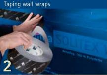
Place TESCON EXTORA centrally over the overlap, unroll and press down over the joint.
