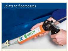
To adhere joints on floorboards, masonry or concrete or other rough substrates, use ORCON joint adhesive. Clean the substrate and apply a continuous bead approx. 5 mm thick (more may be needed on uneven substrates).
