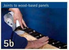
To create windproof joints between wall wraps and smooth, non-mineral surfaces such as wood-based panels or planed wood, place TESCON EXTORA centrally over the joint, unroll and stick down over the joint.
