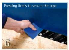
Press firmly to secure the tape, for example using a pro clima PRESSFIX to do the job effectively and to protect your hands.
