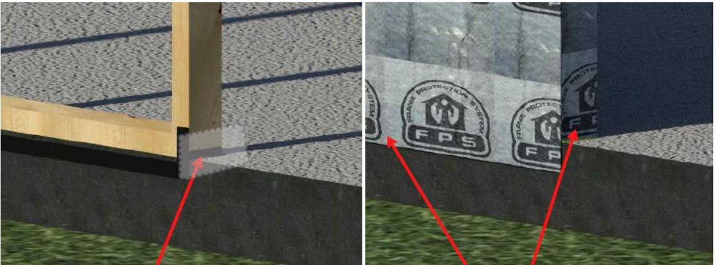
Take a second section of Butyl DS Tape and apply from the outer face of the bottom plate around to the inner face of the bottom plate at the floor line.
