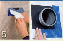
Seal all round penetrations with KAFLEX or ROFLEX grommets.
