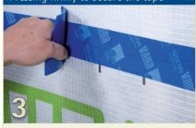
The TESCON VANA tape should be applied centrally and pressed down firmly using the pro clima PRESSEIX
