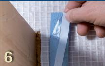
Seal corners using pro clima TESCON PROFIL tape. Remove one strip of the split release paper and press down the first piece.
