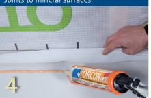
The liquid adhesive ORCON is applied to join the INTELLO® membrane to concrete or wooden frames. Do not press the adhesive bead completely flat.
