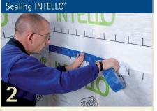
Seal the membranes at overlaps without strain or loading, using TESCON VANA tape.
