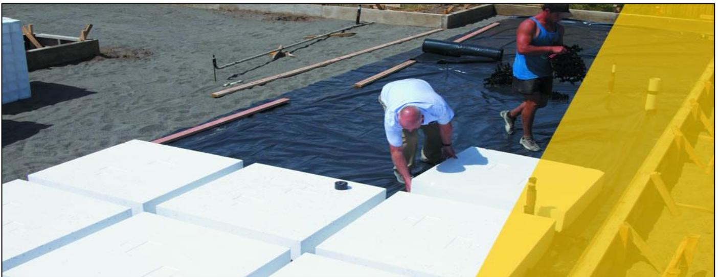
Allied Superslab is proud to offer a greener alternative to the polystyrene pods. Qpod is a recycled plastic dome system which clips together to form a 1100mmx1100mm and 220 deep void former which can be substituted for the polystyrene pods. Refer to section 6.1 for the alternative detailing using the Qpod void fillers.
