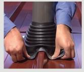
Slide the Roof Boot down over the pipe.
