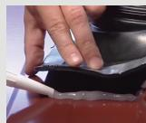
Use self drilling washered screws or sealed rivets to fasten the Roof Boot to the cladding.
