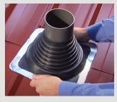
5 Finish by applying at continuous bead of silicone to the edge of the flange and smooth off.
