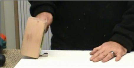
Attach Closet Rail Sockets if needed (tap in, no screws required)
