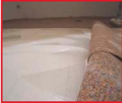
Move to the opposite side and carry out the same process. Once the first strip is complete, move onto the next, adjacent strip ensuring and checking that each strip is tightly butt-joined with no overlaps and NO GAPS. Immediately roll the underlay with a medium weight 45kg stand up roller prior to the adhesive curing. Roll the entire floor in both directions to ensure optimum adhesive transference.
